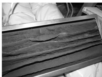
Figure 4 Left: old, dirty building ventilation fan. Reproduced with permission from Steven Lilley, RCPC and RCP. Right: dirty ventilator filter. Reproduced with permission from Professor Tim Sharpe and RCPC.
