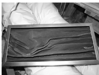
Figure 4 Left: old, dirty building ventilation fan. Reproduced with permission from Steven Lilley, RCPC and RCP. Right: dirty ventilator filter. Reproduced with permission from Professor Tim Sharpe and RCPC.
