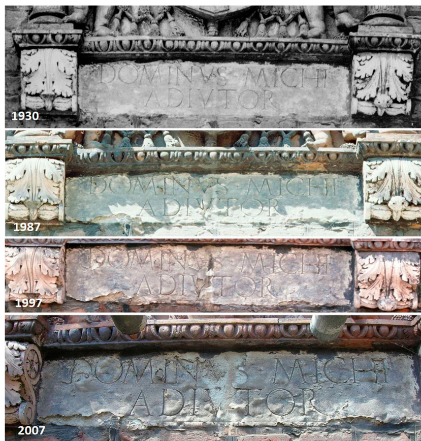
Figure 1. Cardinal Wolsey Plaque at HCP showing acceleration of decay rate on wax-treated Reigate stone surface.
