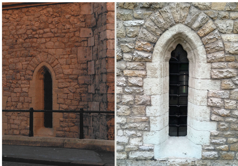
Figure 2. Left: limewashed Reigate stone at Cradle Tower, ToL, shortly after treatment in 1990 and right: in 2018 showing good state of preservation.
