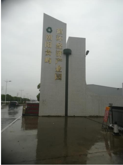
Entrance to the Industrial Park.
