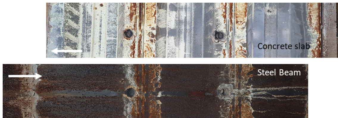
Fig. 6 Stud shearing failure of the 0.9 mm deck specimen at FLS (T2H-1)
