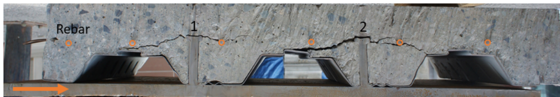
(a) Concrete pull-out failure at ULS (T1-1)
