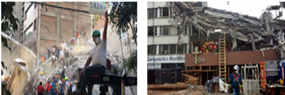
Figure 2. Examples of collapses in buildings surveyed by CICM and SMIE (2017). Other examples are available here: https://notas.tuhogarmexico.com/2017/09/28/asi-lucian-asi-lucen-ahora-los-edificios-se-derrumbaron-en-la-cdmx/
