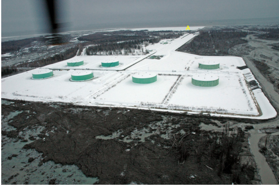
Figure 14. Lahar deposits from the March 22–23, 2009, eruption of Redoubt Volcano that surround the oil storage tank farm at DROT. View is to the southeast toward the shore of Cook Inlet. The main channel of Drift River is left of the tanks. Rust Slough—overwhelmed by lahar deposits—is flowing adjacent to the protective dike right of the tanks; channel modifications directed the main flow of all subsequent lahars down this drainage. The debris in the foreground accumulated nearly to the top of the protective dike, which prior to the eruption was 6 m (20 ft) high. Minor lahar spillage over the dike occurred from flow down Rust Slough (right side of tanks). Point A is the location for the photograph in figure 15 . Photograph by Game McGimsey, AVO/USGS, March 23, 2009. AVO database image at URL: http://www.avo.alaska.edu/images/image.php?id=16985 .
