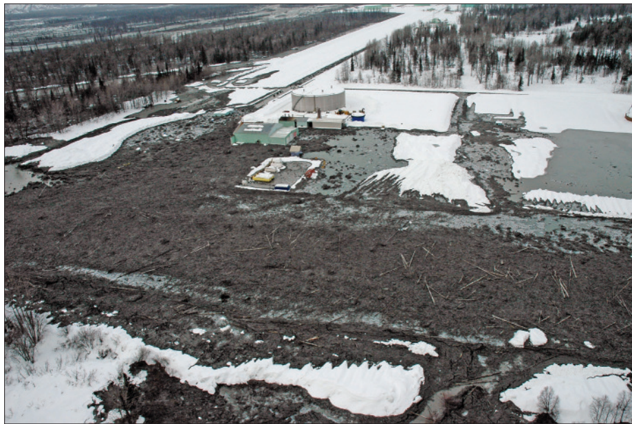
Figure 15. View to the west across the debris-laden airstrip at DROT showing lahar inundation of facilities (up to 2 m, 6.5 ft) resulting from the March 22–23, 2009, eruption of Redoubt Volcano, about 35 km (22 mi) up the Drift River valley. The oil storage tank farm shown in figure 14 is just visible at top of the image. Photograph by Game McGimsey, AVO/USGS, March 23, 2009. AVO database image at URL: http://www.avo.alaska.edu/images/image.php?id=47131 .
