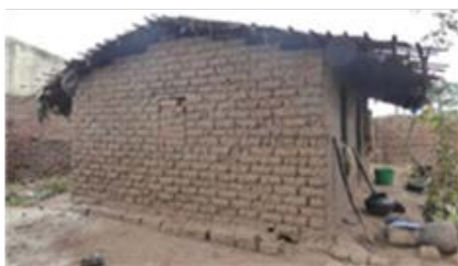
(a) unfired bricks / mud mortar
