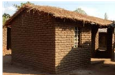
(b) fired bricks / mud mortar
