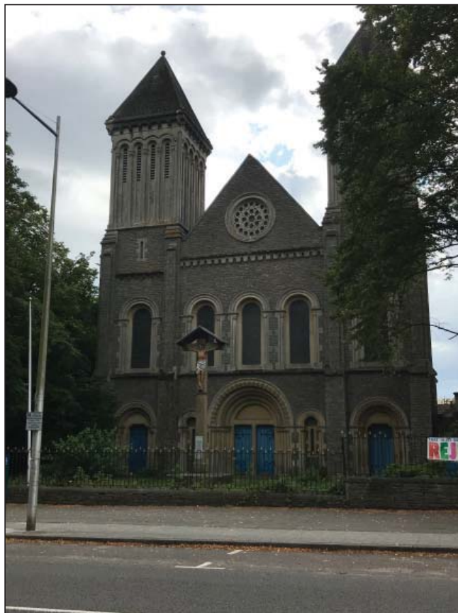
Plate 7 - Church of St. Mary the Virgin, looking west
