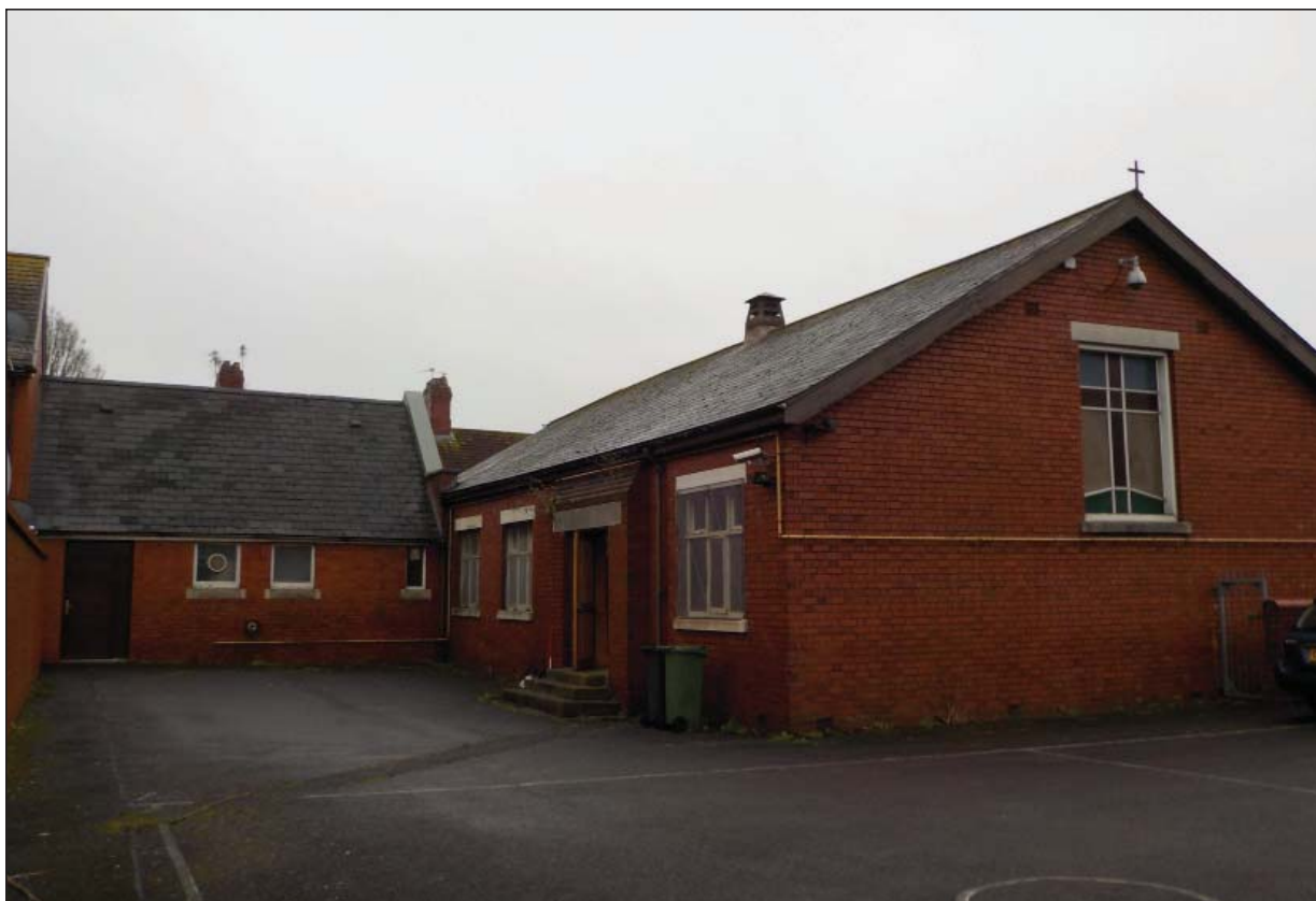
Plate 21 - St. Cuthbert's Church, looking southeast
