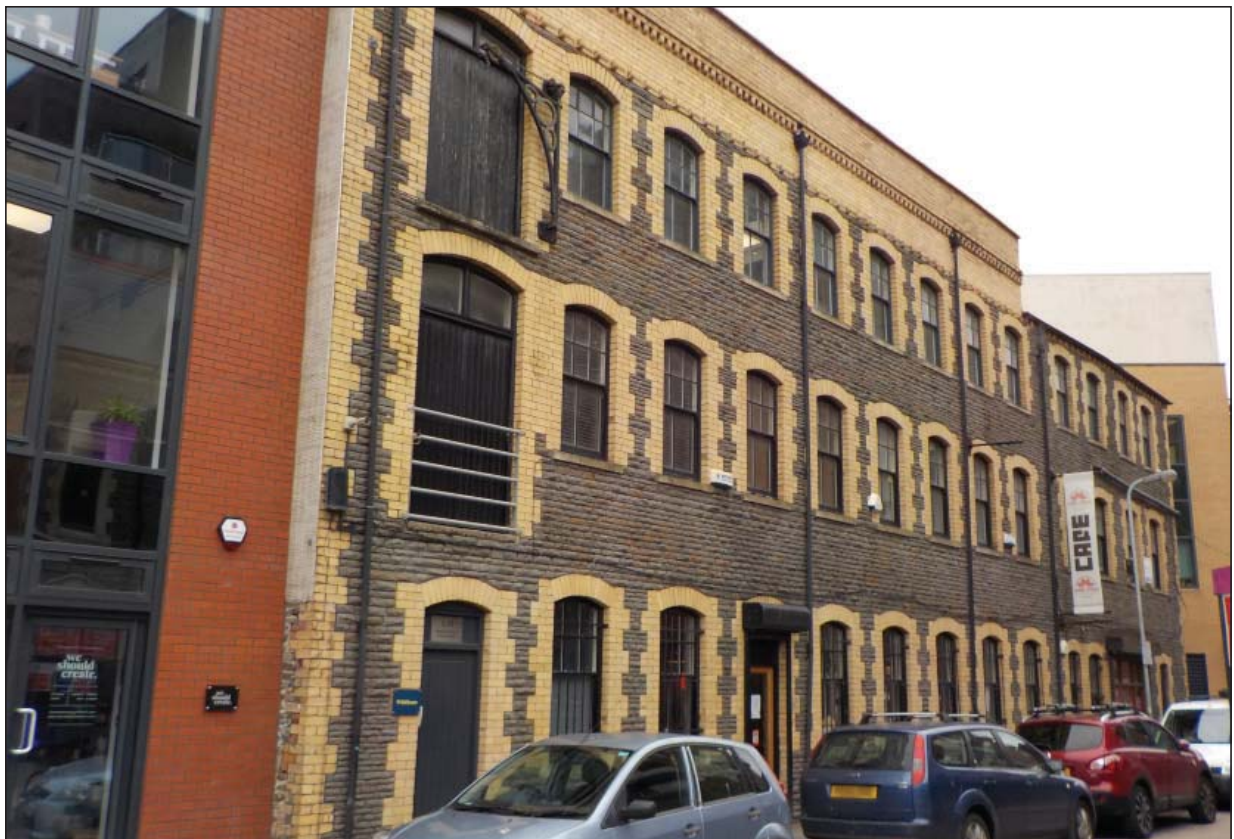
Plate 3 - 2-12 Trade Street, looking northwest
