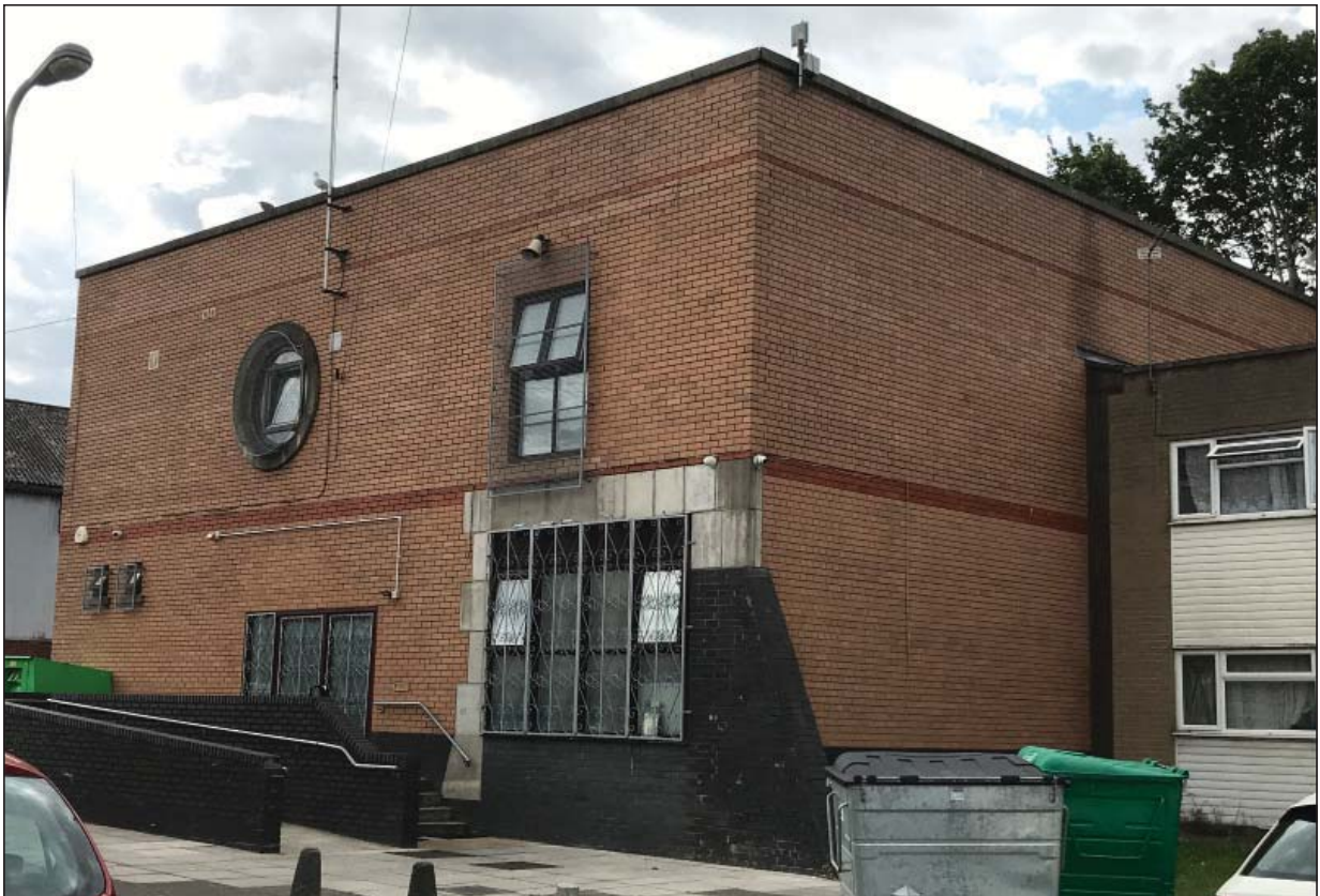
Plate 9 - Noor El-Islam mosque, looking northwest
