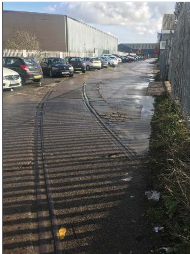
Plate 5 - Rail tracks along Curran Road, looking south
