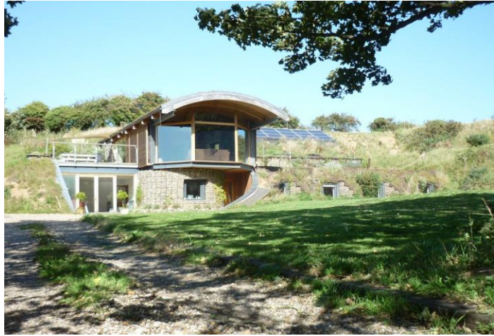
Figure 5: The Sedum House
