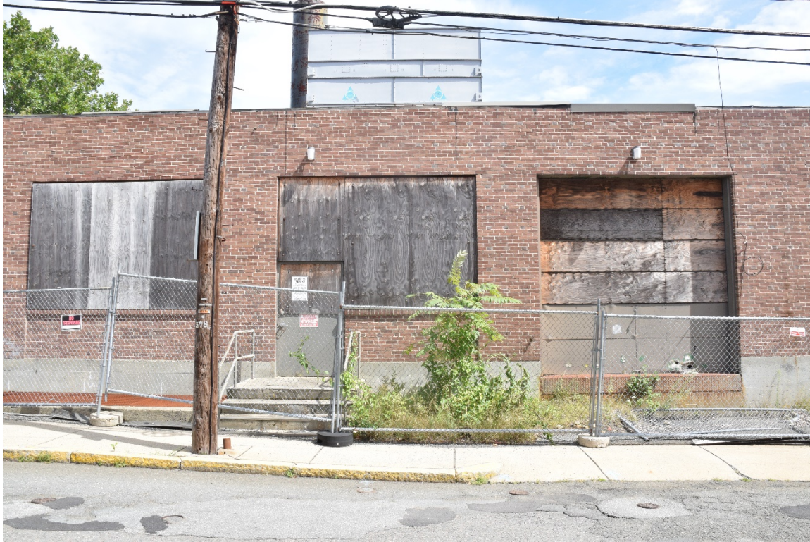
Above: Boarded-up auxiliary building on Hospital Road.
