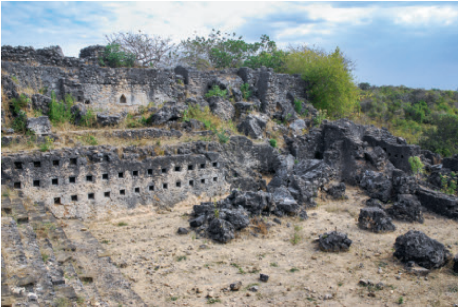
The audience court of the palace of Husuni Kubwa, one of Kilwa's unique architectural gems (photo: S. Wynne-Jones).
