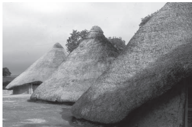
Figure 8. A view of roundhouses 1, 3 and 4; only this view gives an impression of the density of settlement; the area left of this picture is open, and only two other structures stand on the site that should have held 10-12 at any one time; in the background here should have been the defences but they are degraded and make little impact.
