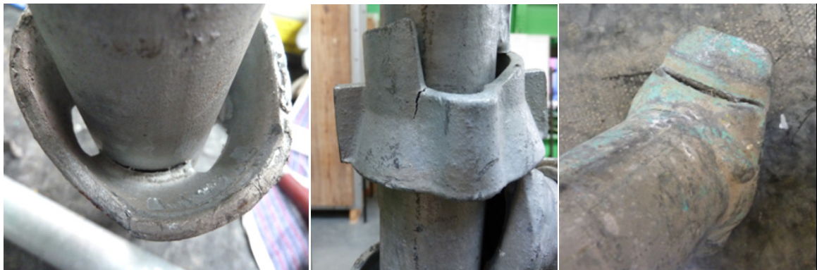
Figure 3.24: Modes of failure. Left: Upward loads, “as new” and used elements, Centre: downward loads and “as new” elements, Right: downward loads and used elements.
