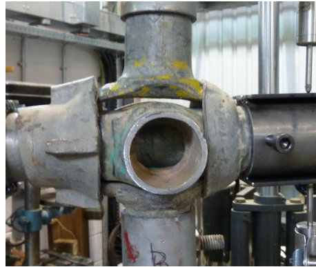
Figure 3.42: Failure at the top part of the joint.
