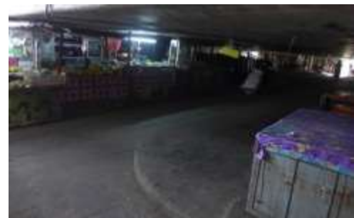
Pedestrian lane under Phaholyothin Rd. bridge (case 3)
