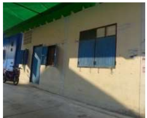
Single storey cement homes
