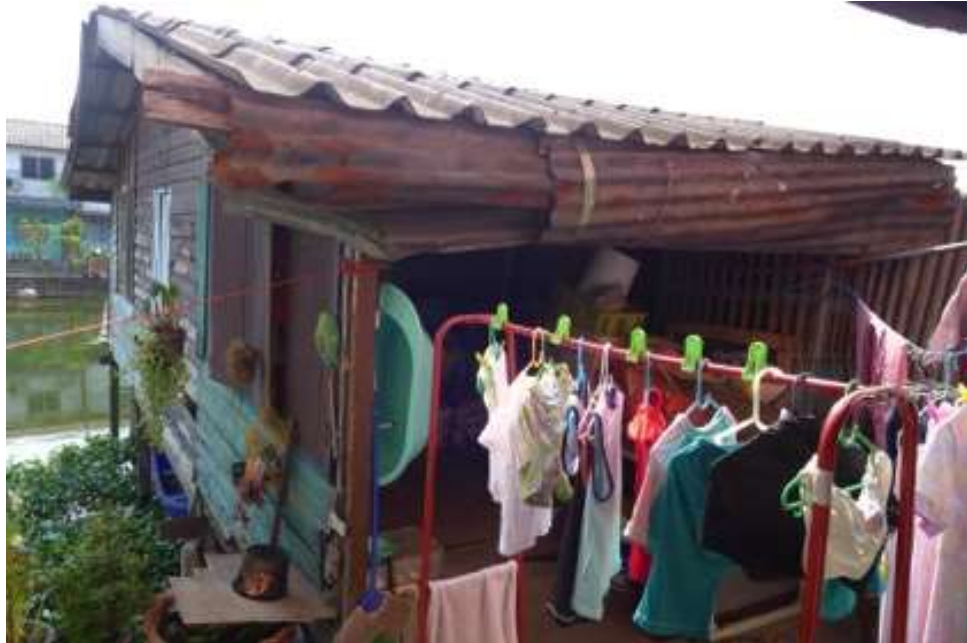
Figure 8.5.1a: A single storey wooden home built on stilts in Saphan Mai neighbourhood. This type of housing is vulnerable to flooding. Source: the author
