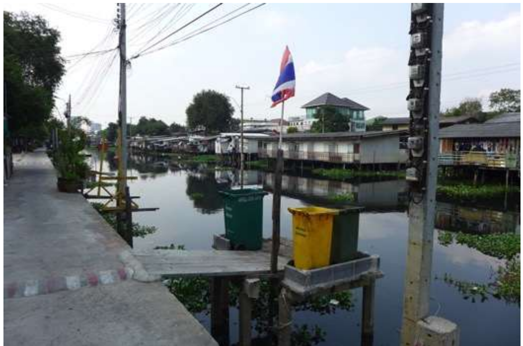
Figure 7.5.2a: Meters for water and electricity (right) monitor consumption for individual households. Source: the author
