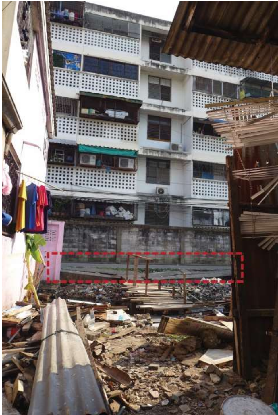
Figure 8.3.1c: A third entrance to Saphan Mai along the backside of an apartment block. Source: the author
