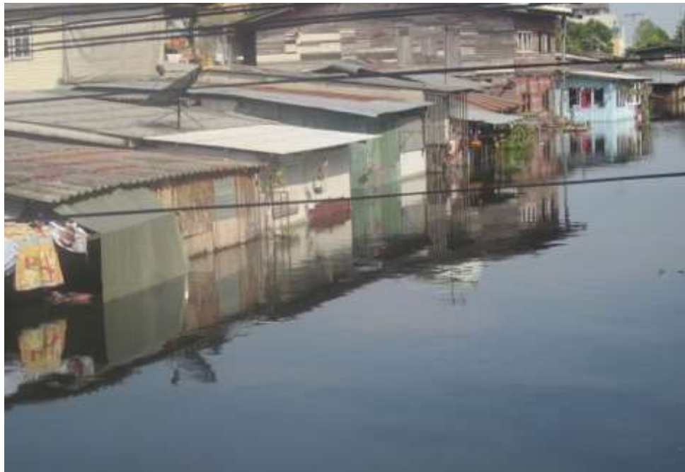
Figure 6.4.1b: The Bang Bua Canal during the 2011. The most vulnerable houses in this photograph are single-storey homes made out of wood and corrugated iron. Single storey homes received a significant amount of damage to their floors, walls and valuable household items that could not be elevated out of the reach of the floodwater. Source: Pattawan Lamjiek
