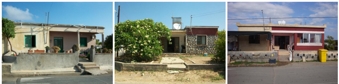
Figure 7.11: Examples of concrete, 'modern' houses, Akdeniz/Agia Eirini.
