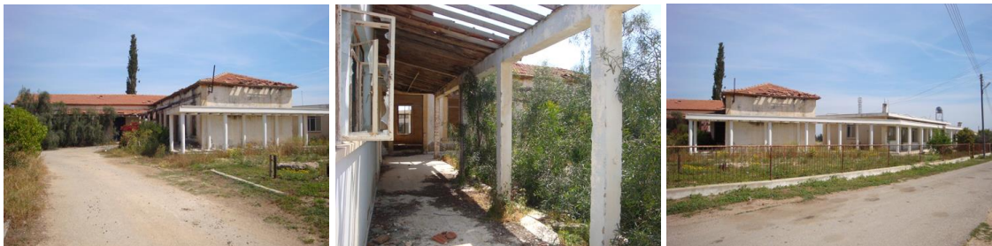
Figure 7.22: Images of the old school building, Incirli/Makrasyka.
