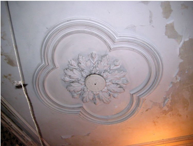
Figure 40 – Traditional Oporto stucco ceiling
