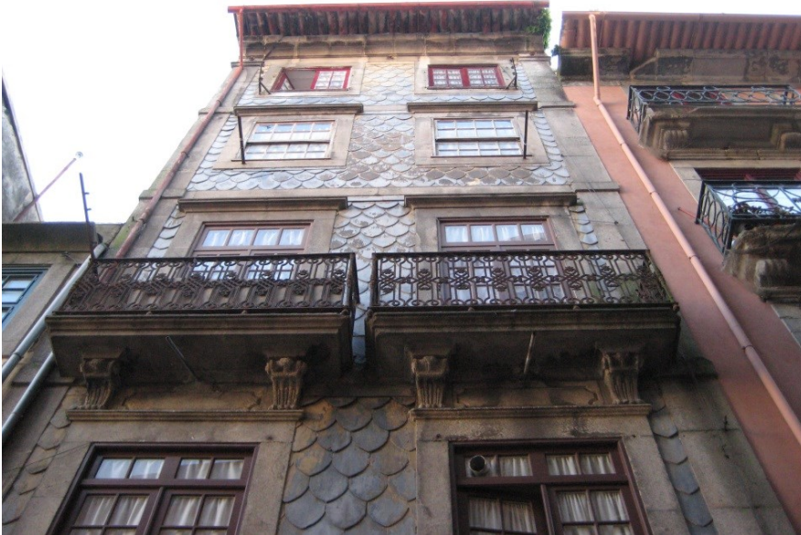
Figure 64 – Case 3 facade with slate tiles cladding
