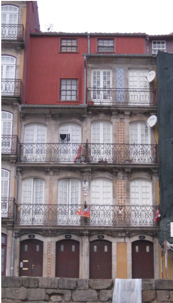
Figure 63 – Case 6 main facade showing the relation between granite mouldings and glazed ceramic tiles
