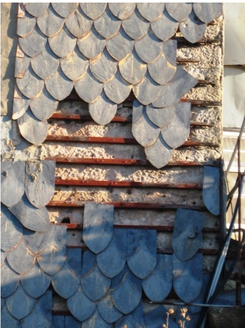
Figure 31 - Slate tiles covering the exterior wall in a ruined building
