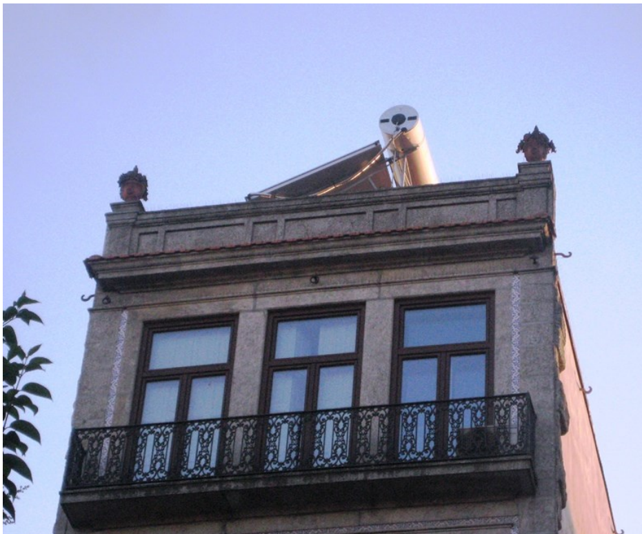
Figure 69 – Traditional building in Oporto with DHW solar thermal panel on the roof (street level view)
