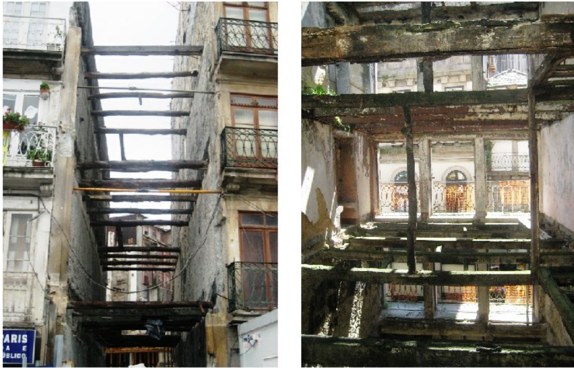
Figure 26 – Wood beams for pavement support in two ruined traditional buildings
