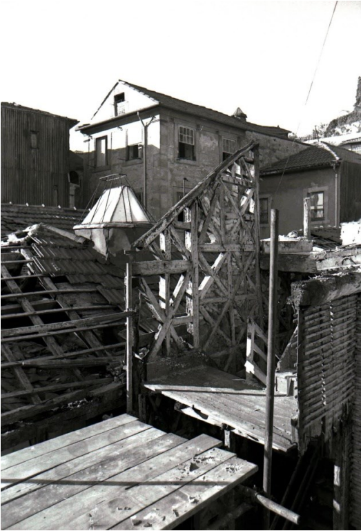
Figure 27 – CRUARB's refurbishment work showing the timber framing construction system (Magalhães, 2010)
