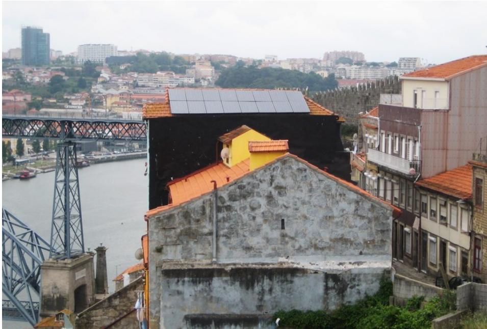
Figure 68 – Traditional building in Oporto with Photovoltaic panels on the roof
