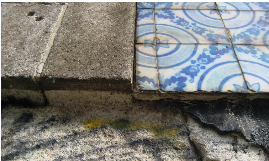
Figure 78 – Windows granite casing in a 19th century traditional building (in ruins) in Oporto
