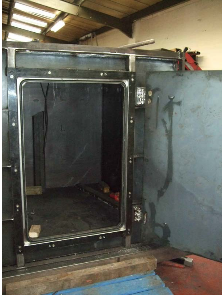
Figure D1.5: Test tank during construction 2
