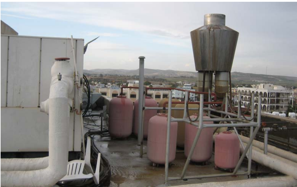
Figure 4.1 Typical view of a hotel roof indicating congested HVAC installations
