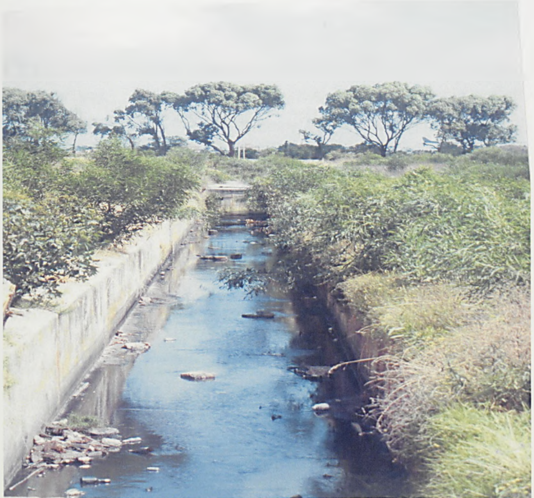
Figure 7: Storm-water canal across the site in Langa
