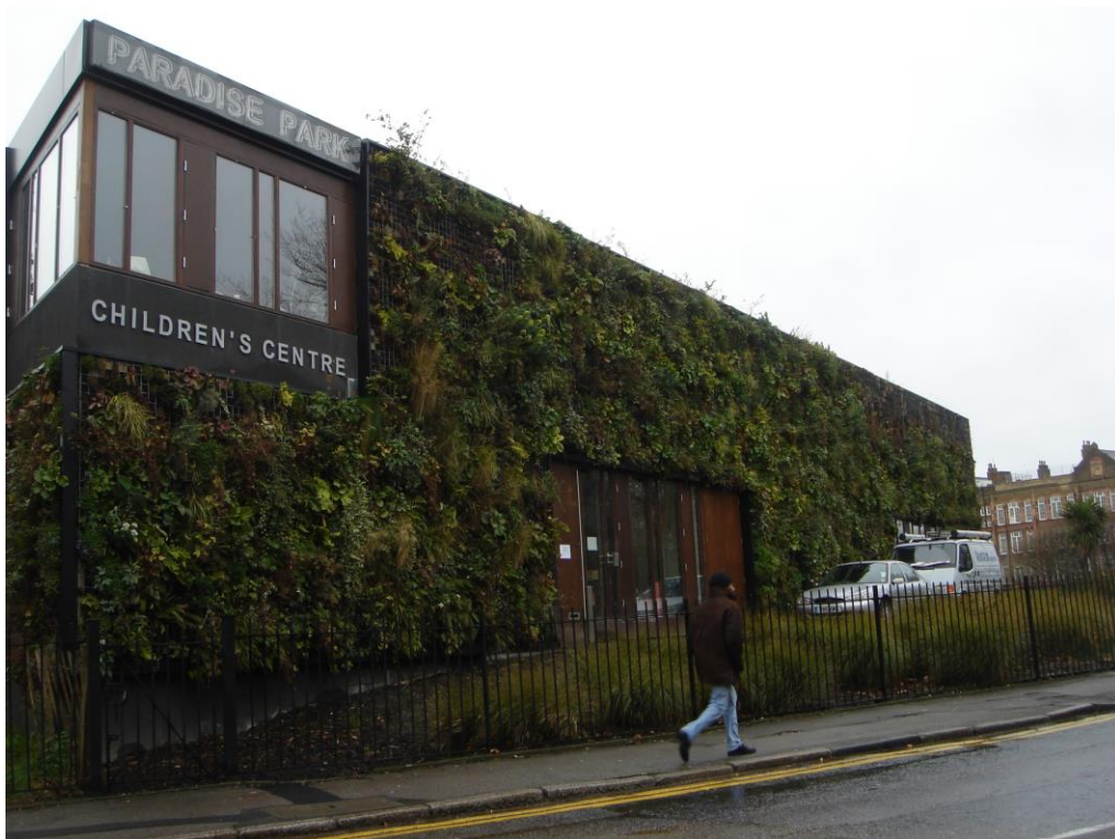
Figure 46: Paradise Park Children's Centre, London (Source: Author)
