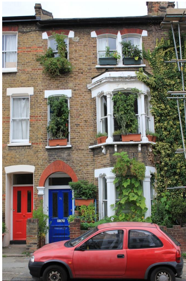
Figure 21: Ridsdill Smith's 5 south facing windowsills and patch of concrete. NOTE: The plants are blocking some glazing area which would reduce the natural light entering the building. This may be beneficial on a south facing and west facing façade during the summer period to reduce over heating but north facing windows would want to maximise light entering through them (Fennel&Fern, 2012b)
