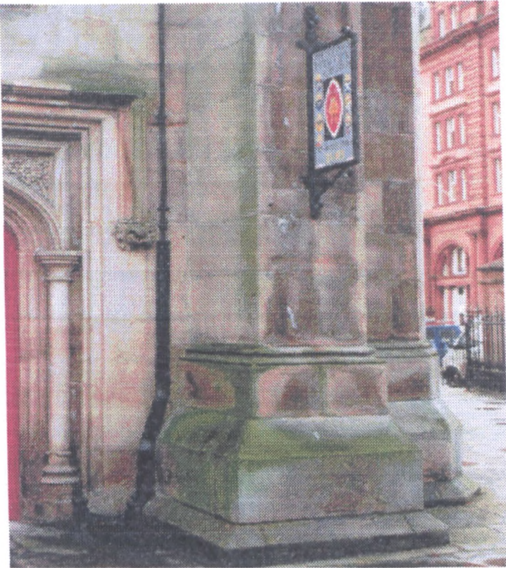
Photo 1.3 Detail of biological colonisation after chemical cleaning at St Mary's Cathedral in Edinburgh.
