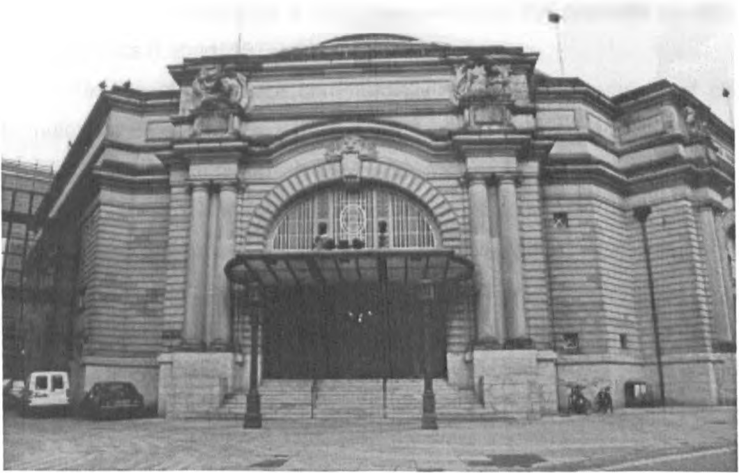
Photo1.1 The Usher Hall in Edinburgh was chemically cleaned in 1996.
