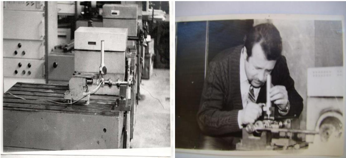
*Puc. 12. The testing machine for fatigue strength tests. Recording of the testing machine indications.*
