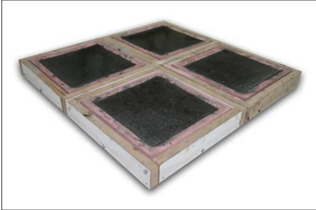
Figure 9.34: Casting Refractory concrete in the Rubber mould.
