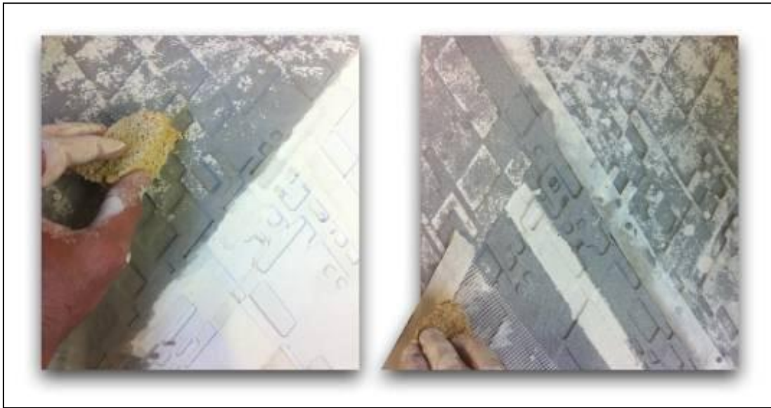
Figure 9.88: Applying glaze with sponge – building up layers and overlaying differing colours.
