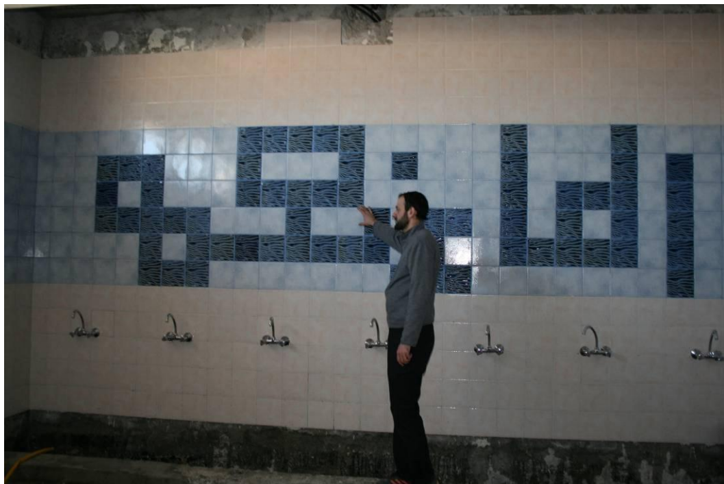
Figure 9.36: Tiles installed in 'Kofic' calligraphy design on the wall of the washing area in the newly constructed Muneerah Al-Saeed mosque (located in Duha City, Kuwait).
