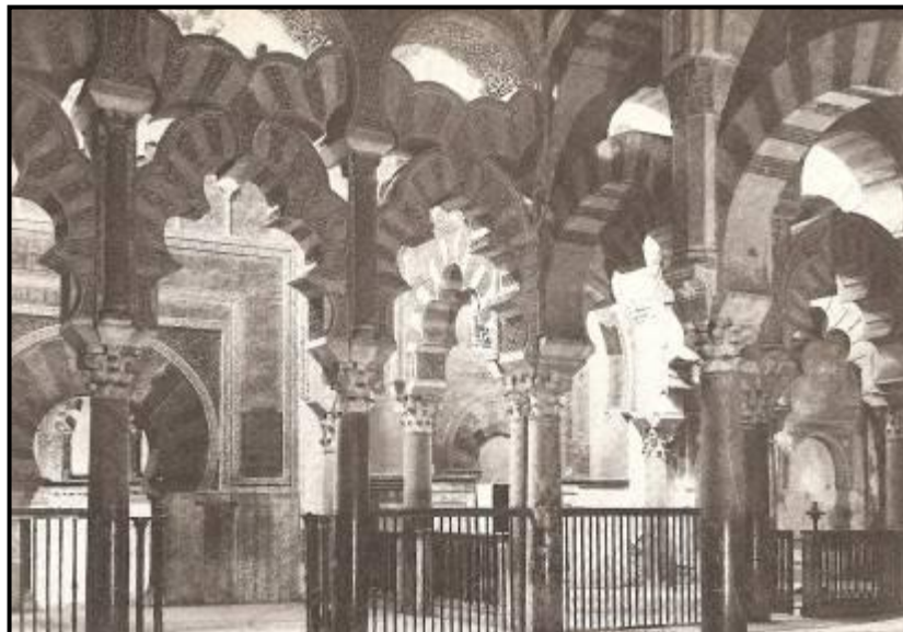
Figure 6. 4: Sanctuary of the Great Mosque at Cordova. The mosque was begun in the eighth century but was frequently added to, especially during the tenth century. The hexafoil arches in two tiers represent a new and original departure in Islamic architecture (Rise, 1975).
