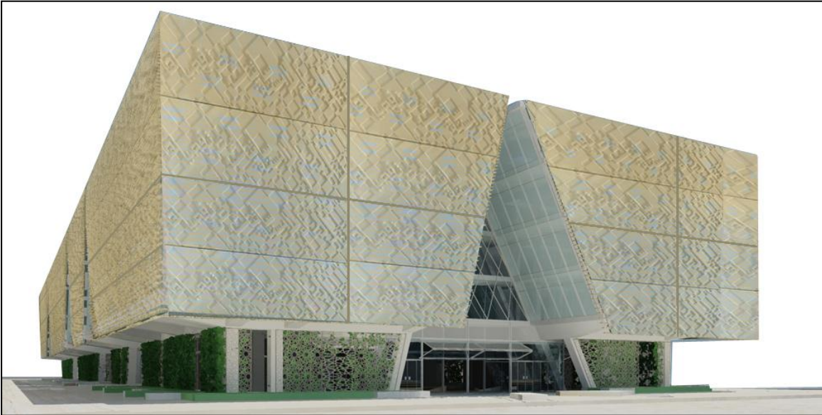
Figure 9.92: Unglazed, relief 'Poetry' tile design applied to building. This effect could be achieved by using cast concrete panels.
