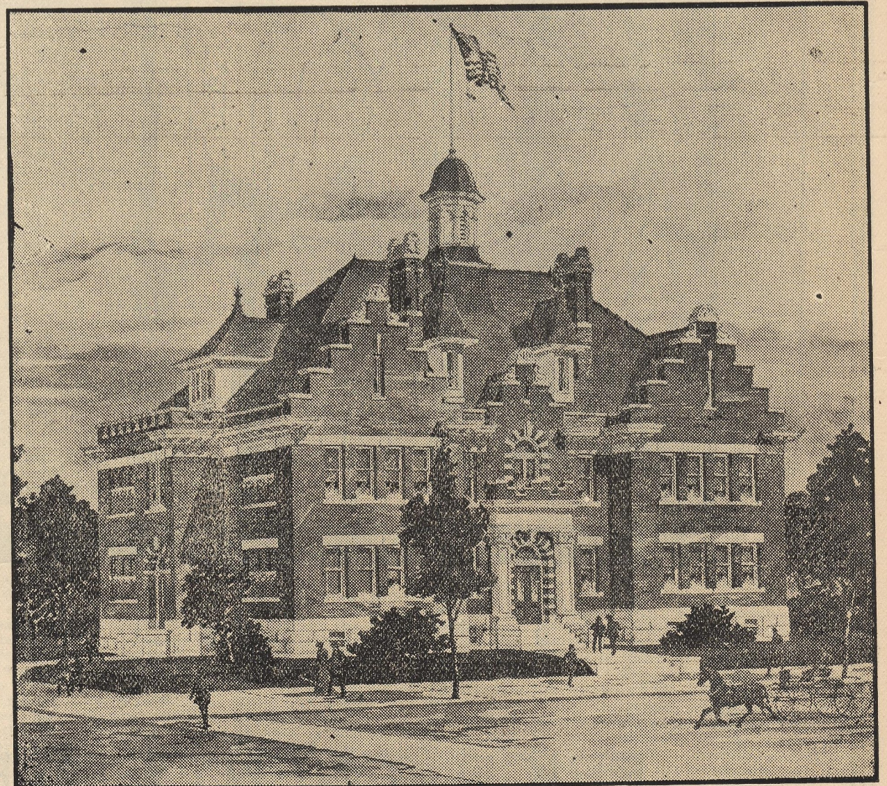
THE CENTER STREET HIGH SCHOOL BUILDING.
