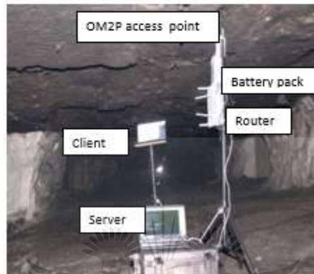
Figure 43: Experimental set up in Bathopele Platinum Mine tunnel
