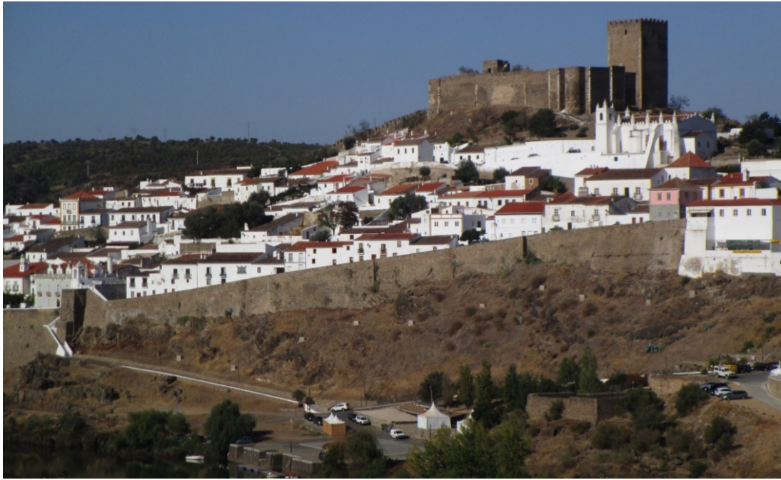
Figure 2. View of the town of Mértola from the left bank of the Guadiana river. The wall, the Mother Church, and the castle can be observed.
