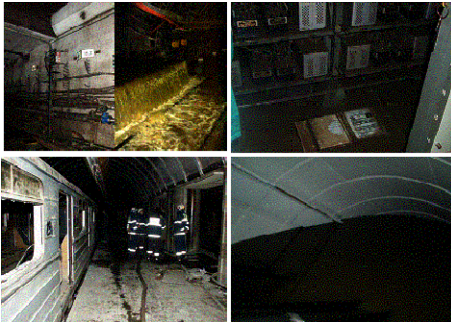
Figure 4.4: Damage in the Prague Metro Photos from http://tom.vlakpage.cz/index.htm
