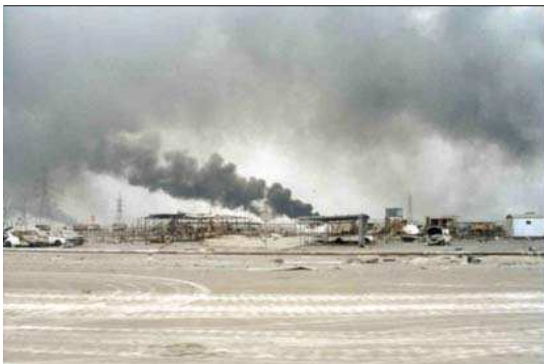
Figure 13. Destroyed oil installations in the Burgan Oil Field, April 1991.
