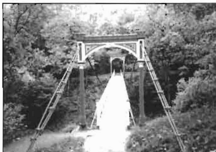
Image 4: Restored bridge in the town park
