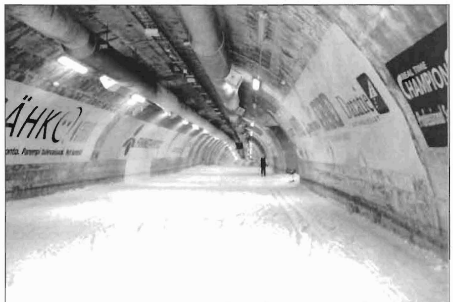
Image 8: Skitunnel in Sotkoma, Finland
