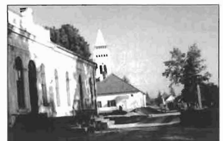
Image 7: Construction works beside the manor
