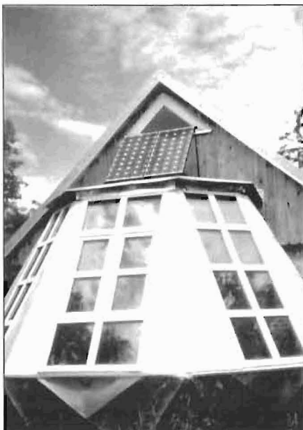
Image 8: Sun dome with photovoltaic panels
