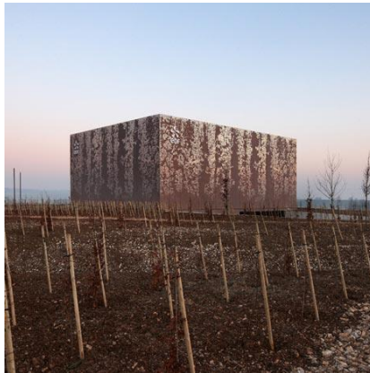
Figure 2. National archives of energetic company EDF building, France. 2011. Architects: LAN
