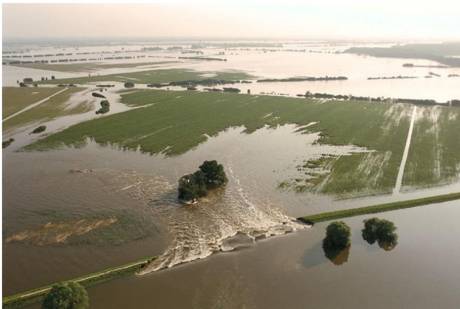
Figure 2: Flood August 2002 of the Elbe river with a dyke breach, Germany © André Künzelmann/UFZ (Arnhold 2008).
