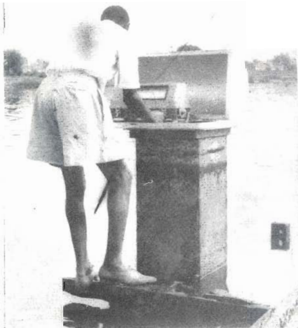
Lake level recorder at Kisumu on Lake Victoria
