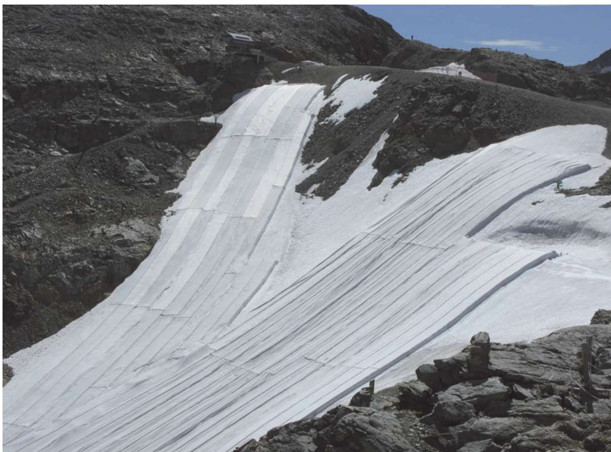
Fig.: Blanketing the Bernina Group Glacier in Summer – Adaptation to Climate Change Impact.
