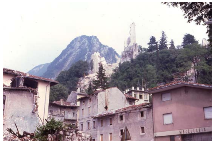
Fig. 1: Damage in Gemona di Friuli Caused by the 1976 Friulian Earthquake.
