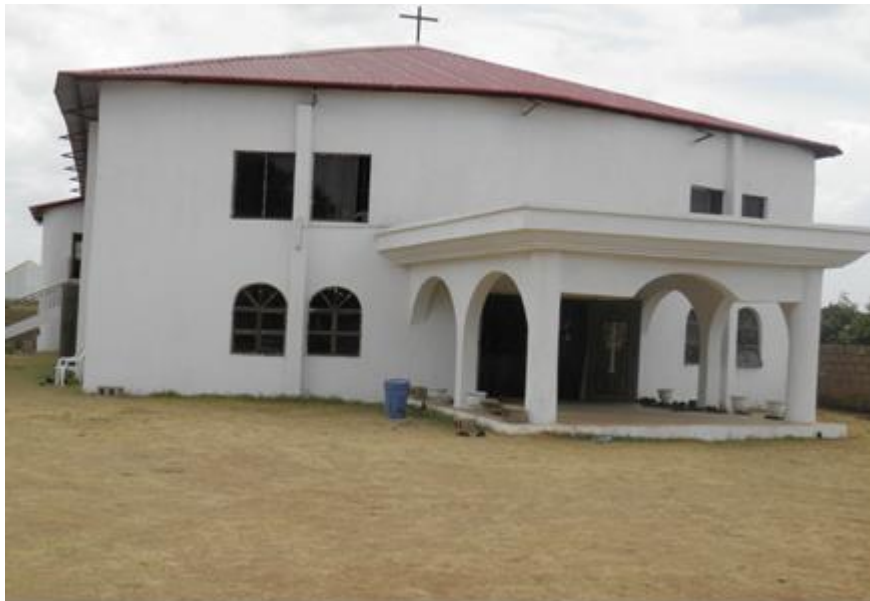
Figure 35. Front view, CSMC, Ray Field, Jos. Photograph: T. O. Baiyewu. May 2013
