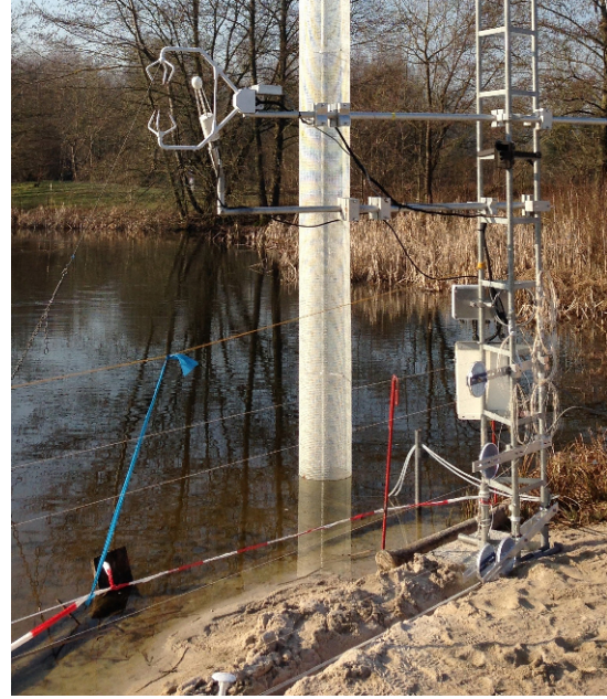
(b) final installation of CSAT and LICOR at the lake after extension of the mounting for flux measurements above the lake
