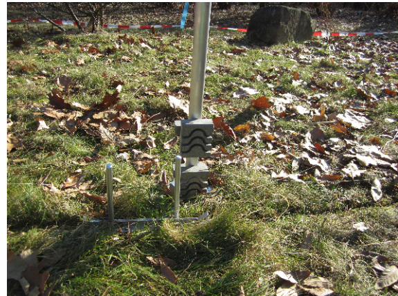
(b) Plow inserted into the ground
