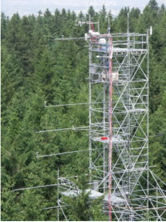
Main tower M1
