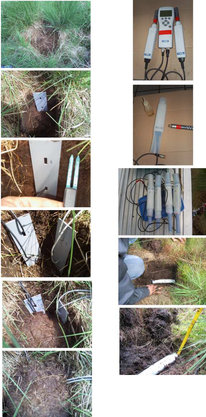
Figure 3. Installation of moisture, temperature sensors (left) and CO 2 sensors (right).
