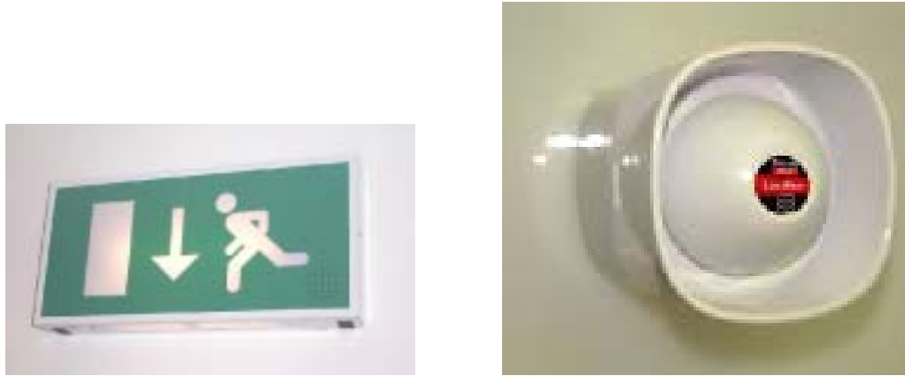
Fig. 5.7. Directional sound is based on sounders (right) that are integrated in the exit signs and allow sort of an intuitive orientation based on sound beacons.
