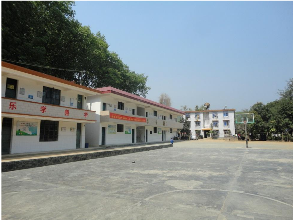
Image 5: Schoolyard and newly renovated school building of one visited school.
