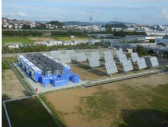
1 MW/5 MWh VRB - Sumitomo - Japan
