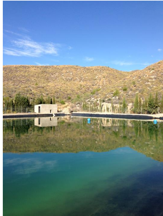
Plate B. Purpose build reservoir
