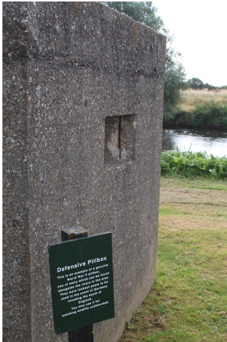
Figure 2. Pill box incorporated into the memorial landscape beside the River Trent. Photograph: Howard Williams, September 2012.
