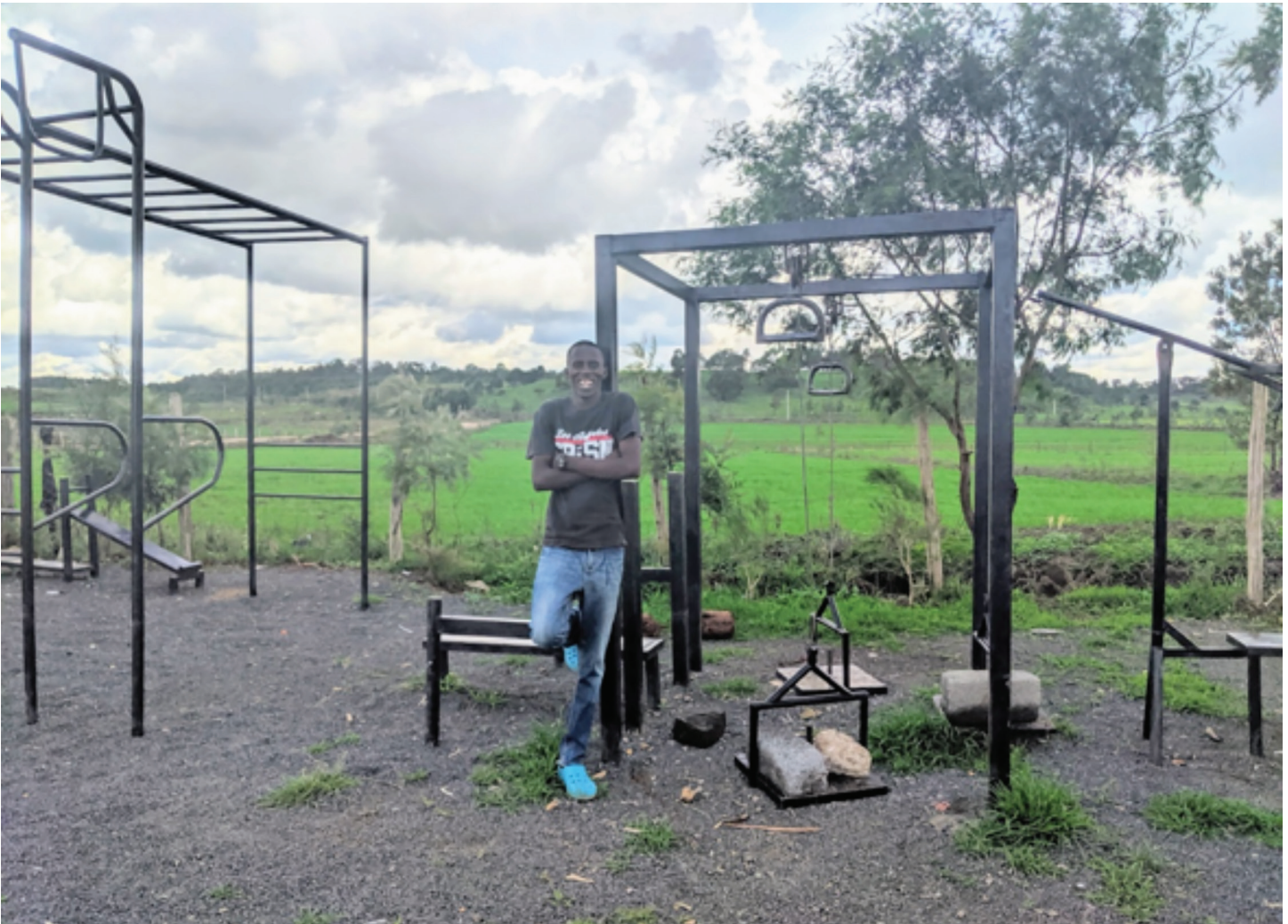
Figure 3. The second author at the completed outdoor gym.
