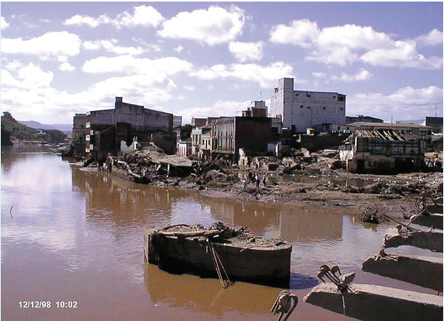
Figure 2. This photo, taken in December 1998, shows the destruction that Hurricane Mitch caused in Tegucigalpa, Honduras's capital. Photo credit: U.S. Geological Survey.
