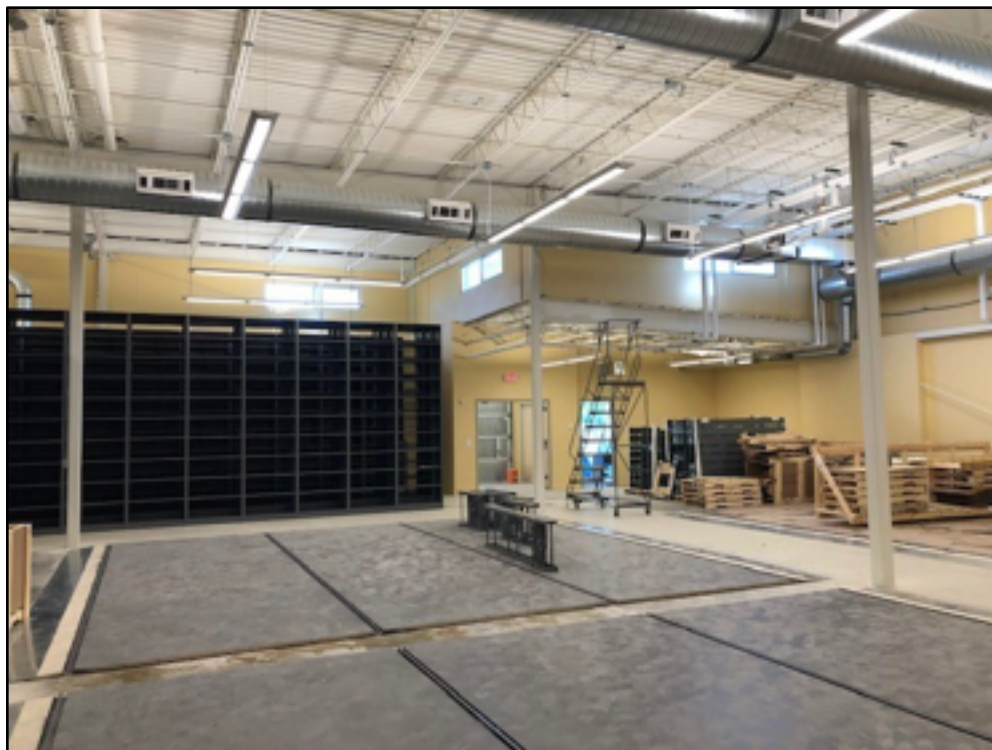
Figure 1. The future Library Annex undergoing renovations. Photo credit: Rachele McLain.
