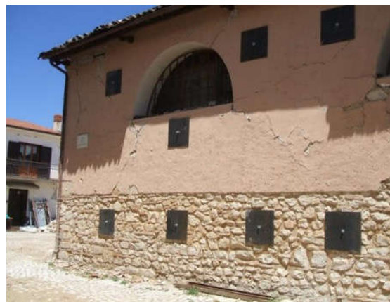
Figure 9. Stonework building in Onna, near L'Aquila in Italy: the arrangement of the stonework is uniform, and the masonry texture is well-organized (homogeneity of the stones and random presence of bricks to improve the overall wall's stability) (combination No. 12, Table 4). It can be noted that this wall was consolidated using a deep repointing the mortar joints. The medium dimensions of some stones suggest a good connection between wall leaves. The masonry material of this building did not disaggregate during the 2009 Aquila earthquake. It should be also highlighted here that most historic masonry buildings of Onna, typically made of a masonry of lower quality, disaggregated during the 2009 earthquake [28].
