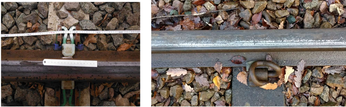
Figure 9 Leaf layer transfer down the railhead (left), leaf layer as encountered in the field (right).
