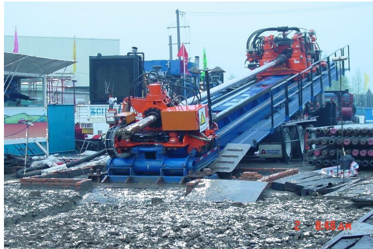
Figure 2-2: Drilling rig system.
