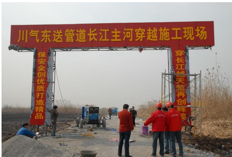
Figure 4-1: Construction site of Yangtze River main channel crossing project.
